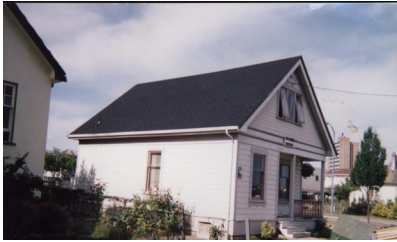
The original Anawim House...
