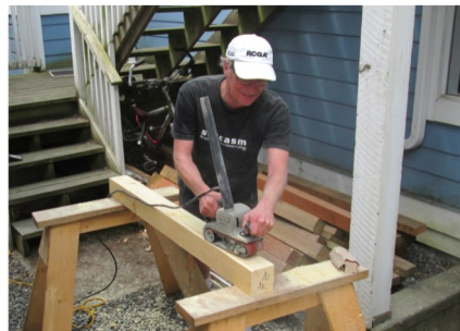
Daniel sanding the rough edges off the fence posts
